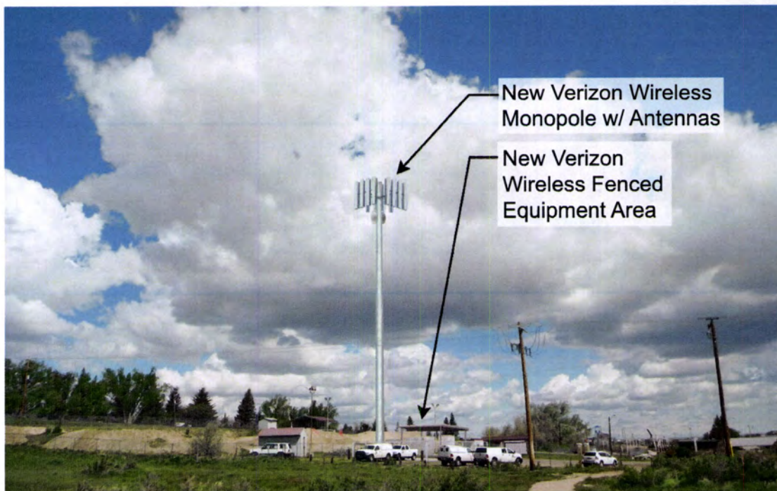
New Verizon Wireless Monopalm w/ Antennas & Equipment Compound
